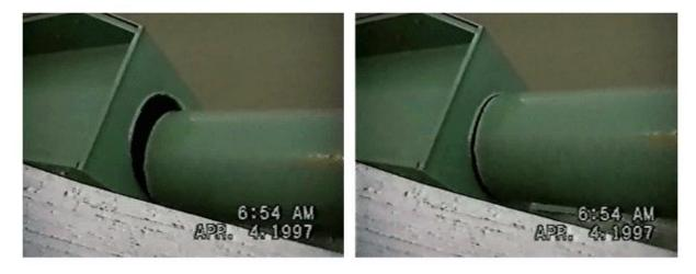
Figure 1.8 Broken Guide Pipe – Fred Hartman Bridge [11]
