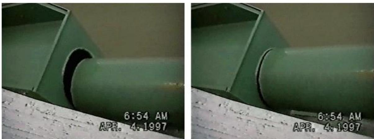
Figure 1.8 Broken Guide Pipe – Fred Hartman Bridge [11]
