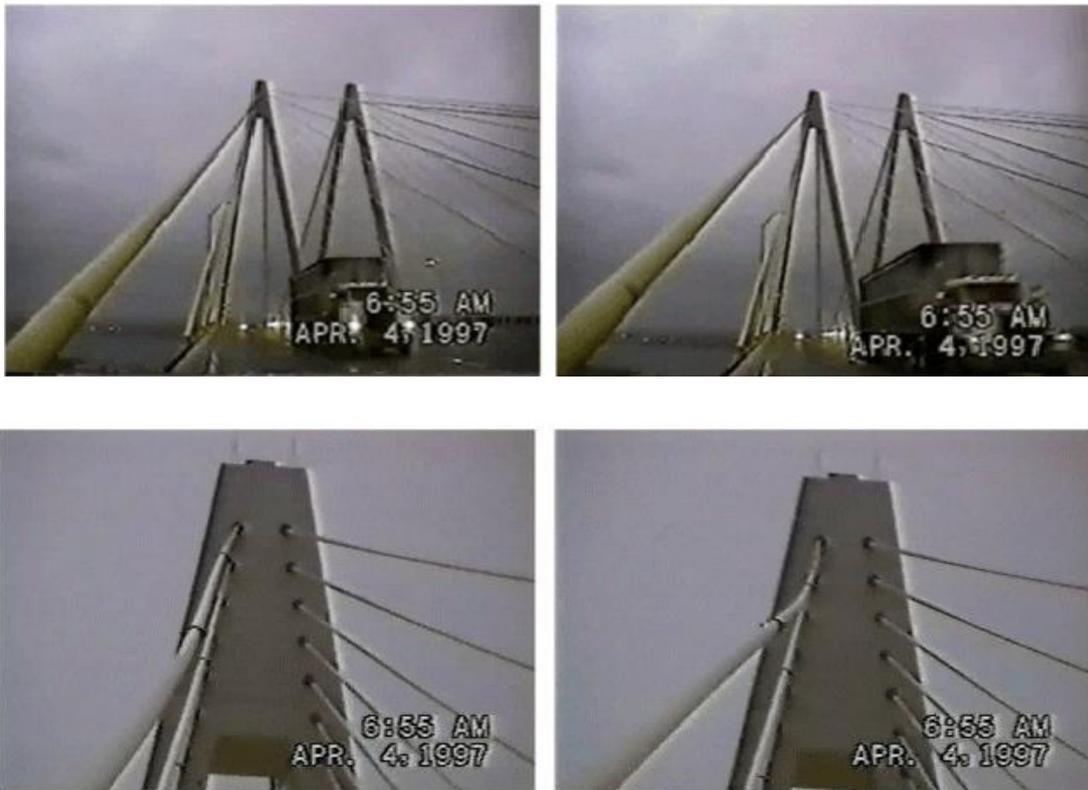
Figure 1.7 Recorded Rain-wind induced vibrations on cable stays: Fred Hartman Bridge [11]
