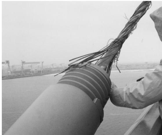
Figure 1.3 Damaged stay cable at the lower anchorage [9]
